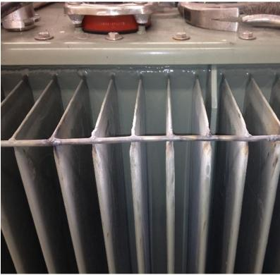
These repairs are done on site without draining oil (fast and minimal loss of production)
